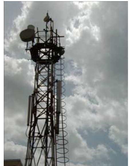
Typical Aircel/DWL deployment of Alvarion BreezeMAX base station
